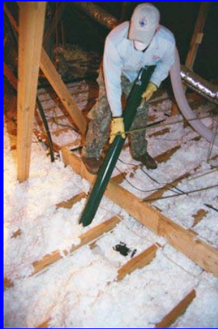
Removing Contaminated Insulation
